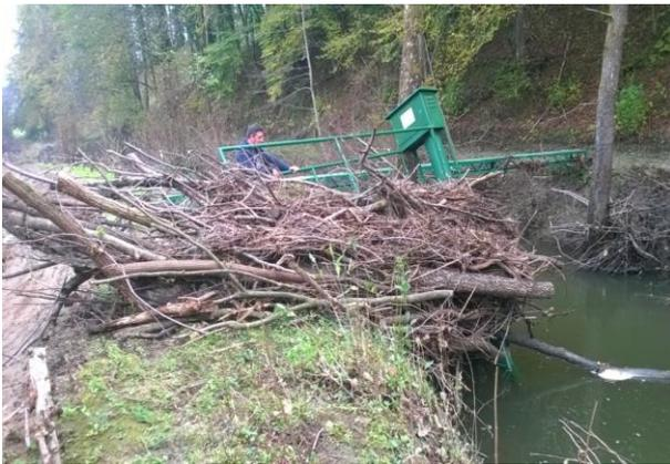
*Figure 32 Soil erosion and debris flow destroyed the GS Trepča - Traverza, during the 2014 flood*
