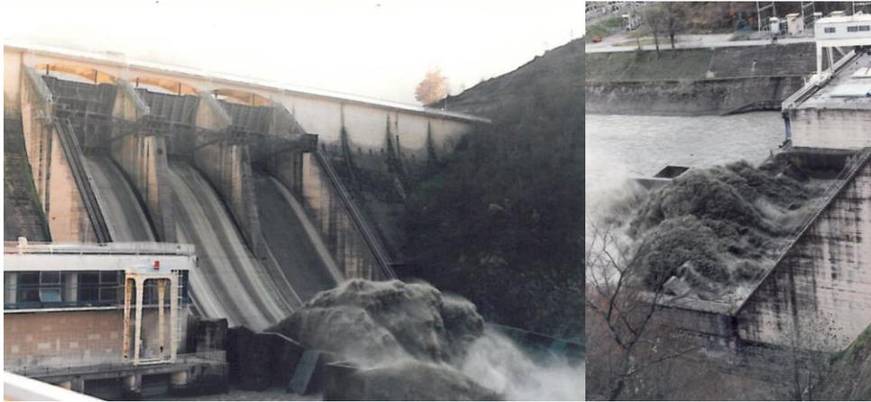
*Figure 29 Discharge from the bottom outlets of the HPP Potpeč in 1999*
