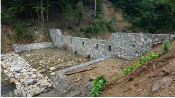
*Figure 34 Sediment retention dam in the Jadar River Basin*
