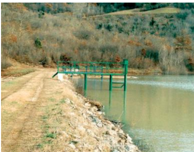
Figure 86: Water-level recorder (limnograph)
