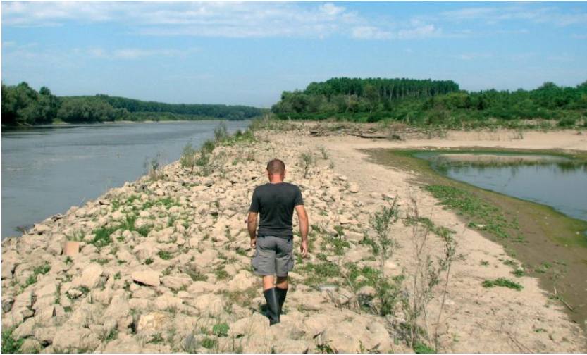
Figure 5: First guide bund on the Sava River.
