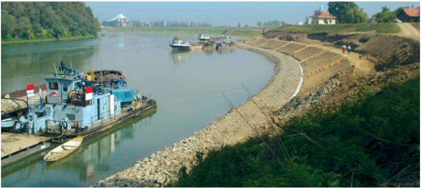
Figure 4: Sloped revetment with crushed stone cladding.
