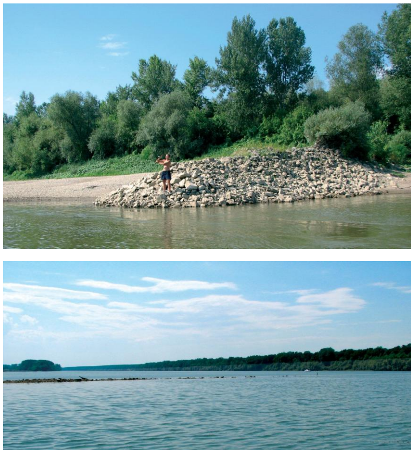
Figure 6: Groynes on the Sava River – Rača sector (top) and Skela (down)
