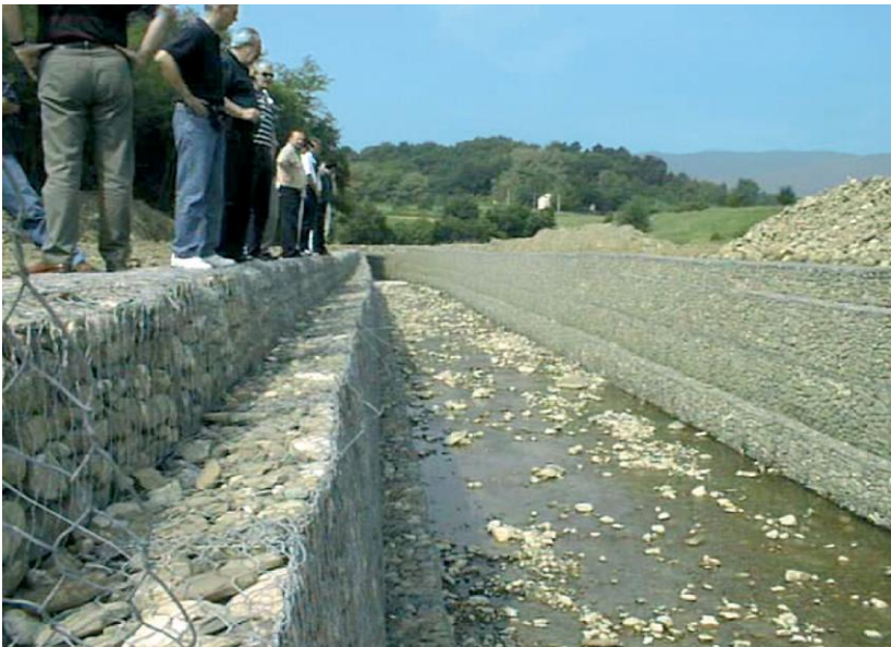
Figure 3: Vertical gravity-based revetment made of gabion mattresses / baskets
