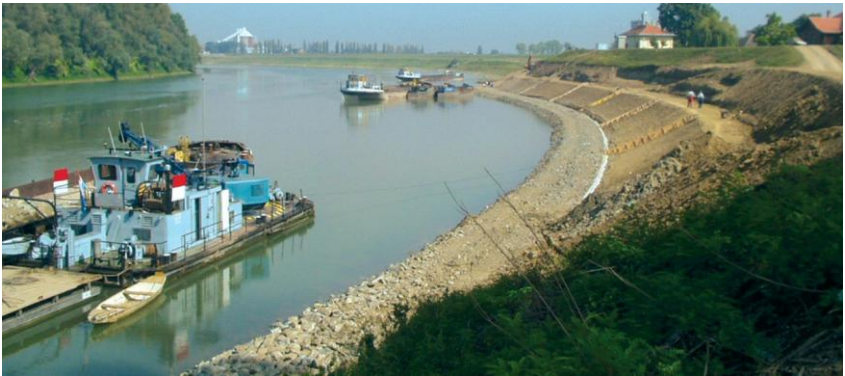
Figure 4: Sloped revetment with crushed stone cladding.
