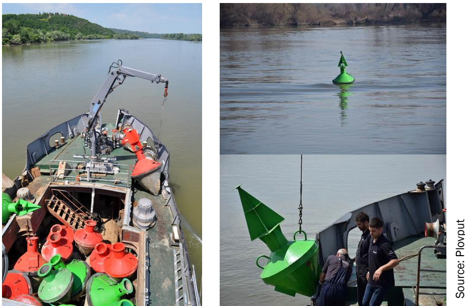
Figure 45: Fairway marking works performed by the staff of Plovput on the Serbian Danube
