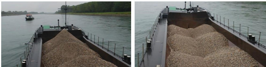
Figure 55: The surveying vessel leads the way to the exact placement spot (left), the hopper barge is opened to release the material (right) (© Katja Rosner, via donau).
