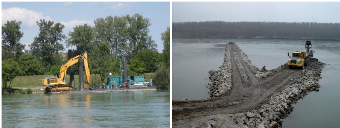
Figure 2: Maintenance works and groyne adaption on the Austrian stretch of the Danube (free-flowing sections Wachau and east of Vienna)
