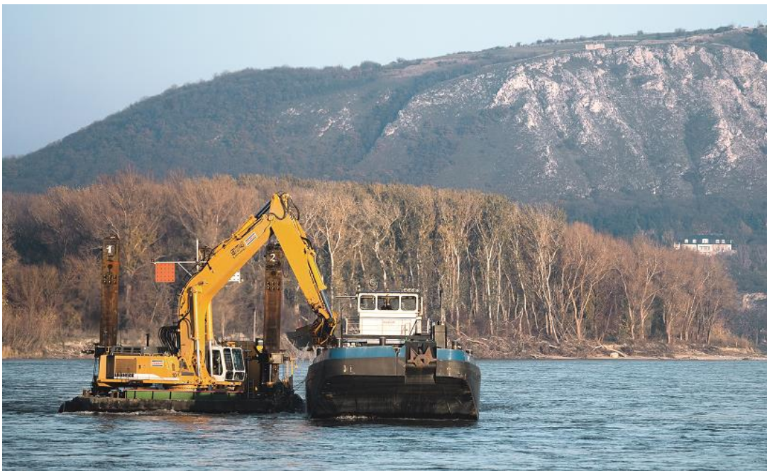
Figure 40: Dredging pontoon with visual signals (floating equipment at work, protection against wash, fairway clear on one side) and hydraulic crane together with hopper barge for transporting dredged sediment
