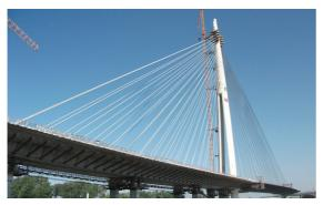
Considering the main span as well as the height (lower edge of the bridge structure is 16 m above the high navigable level), the bridge does not pose a threat to the safe water transport on the Sava River.
