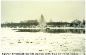
Figure 5. Breaking the ice with explosive on the Sava River near Ruščica (Sl. Brod) - January 17, 1985
