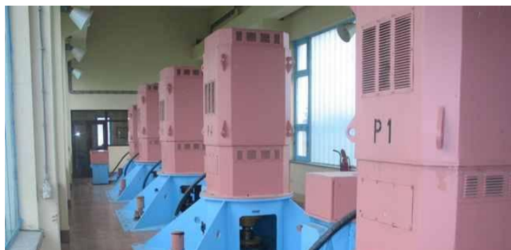
Figure Ap1-3: Flood protection pump station machine room
