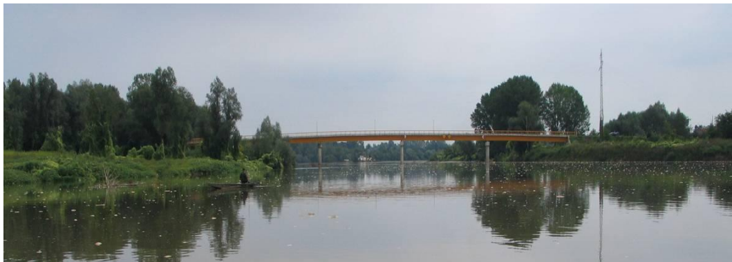
Figure Ap1-17: Bosna River (mouth into the Sava River – bridge in Šamac)
