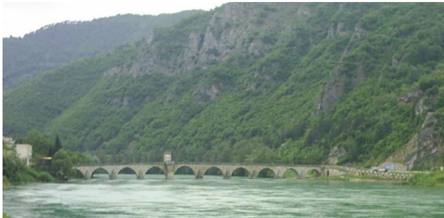
Figure Ap1-21: Višegrad (Mehmed Paša Sokolović Bridge, under UNESCO protection)
