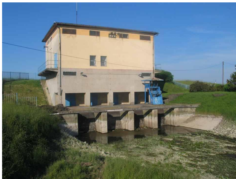
Figure Ap1-5: Pump station structure Liman (Lijevo polje)
