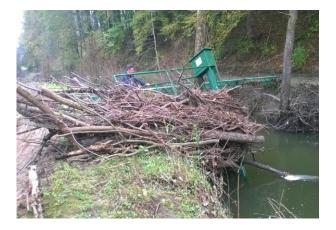
Figure 32 Soil erosion and debris flow destroyed the GS Trepča - Traverza, during the 2014 flood
