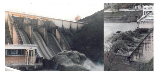
Figure 29 Discharge from the bottom outlets of the HPP Potpeć in 1999
