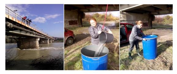
Figure 16 Integrated 200 litre water sample at gauging station Sava-Podsused
